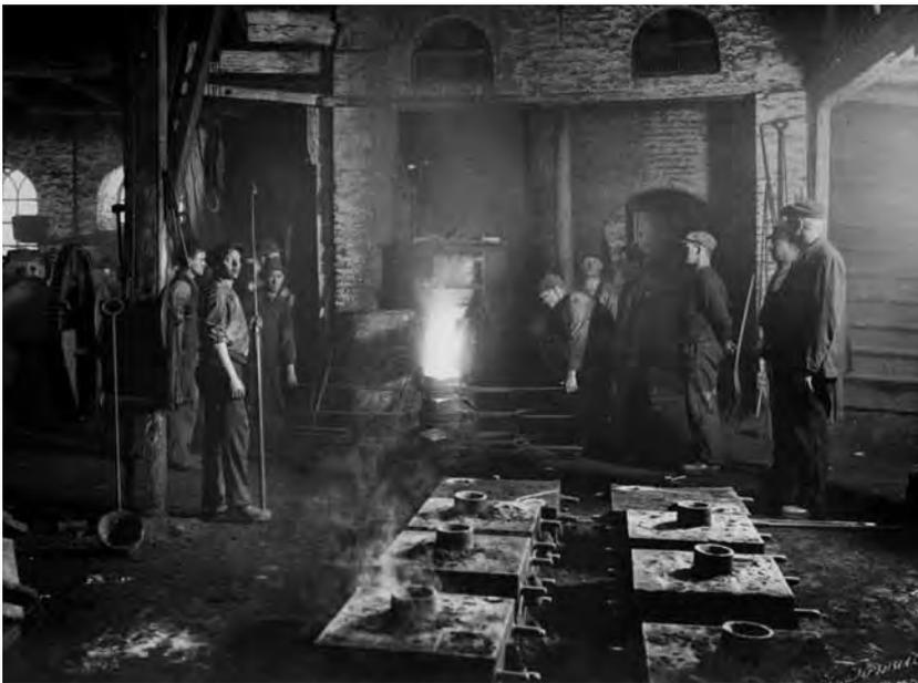
*Moulders and workers are waiting for liquid cast iron to come out of the furnace. They are ready to mould the cast iron just as people have done for 100 years in these buildings.*
