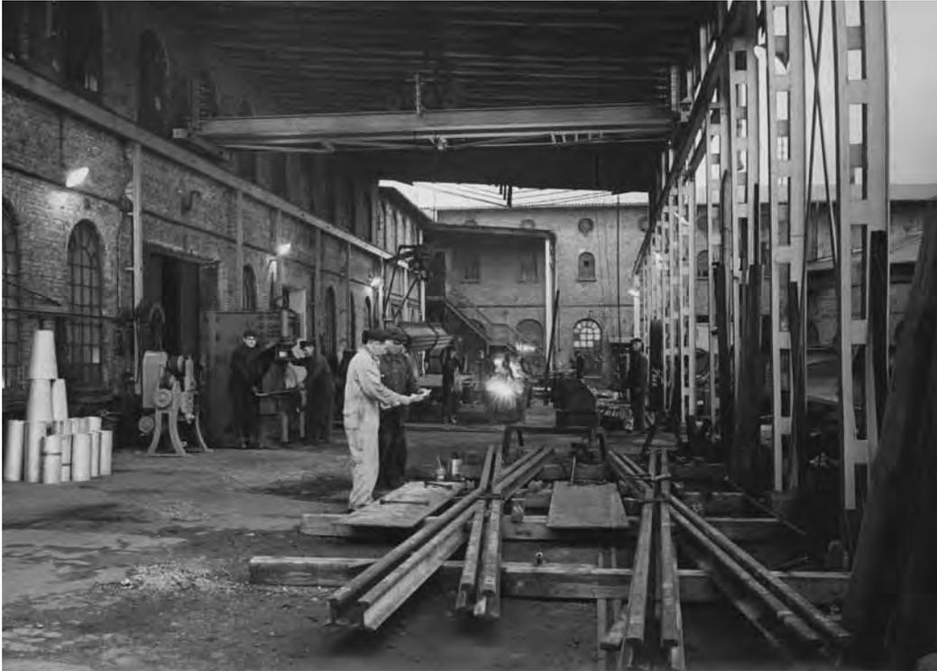
Outside the boiler workshop at De Smithske the large steel constructions were made under a shed roof. Here rail lines for the Danish state railways. Photograph by Clausen, 1960.
