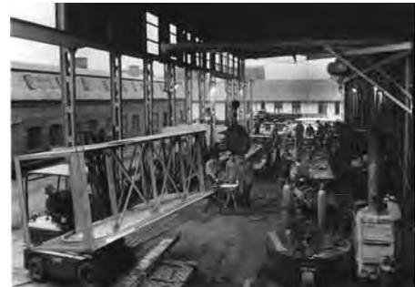
*It was impossible to make large steel constructions indoors so they were finished outdoors in an open shed. The administration building can be seen in the background. From 1970 the division was expanded to include parts of the cement factories 'Norden' just west of De Smithske. However, at the same time the factories in the city disappeared – and so did the orders. Photograph by Clausen, 1958.*
