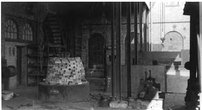
*The casting of church bells has not changed since the middle ages. Each church bell is unique with an individual form and sound. Hence, church bells cannot be produced in batches and production was stopped as church bells only made up 2% of the total turnover. This photograph shows a bell in its mould.*
