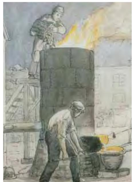
*Cupola furnace at Henning Smith's foundry. The pig iron and furnace coke are added from the top. Air is blown in from below on the left, while liquid cast iron is drawn out on the right. Water-colour from 1871.*
